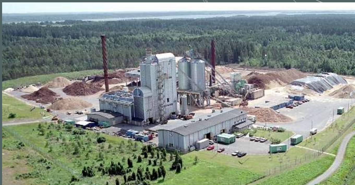
Figure 5.3: Värnamo BIGCC Plant, Sweden
