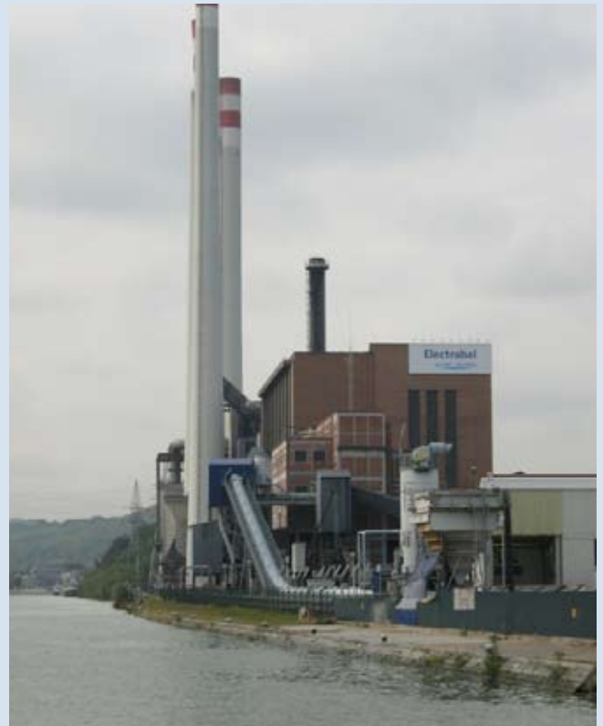
Figure 3.4: Les Awirs Power Station in Belgium
