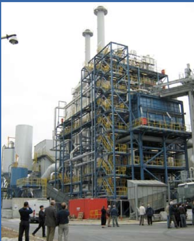
Figure 5.9: Wanze Biorefinery Boiler
