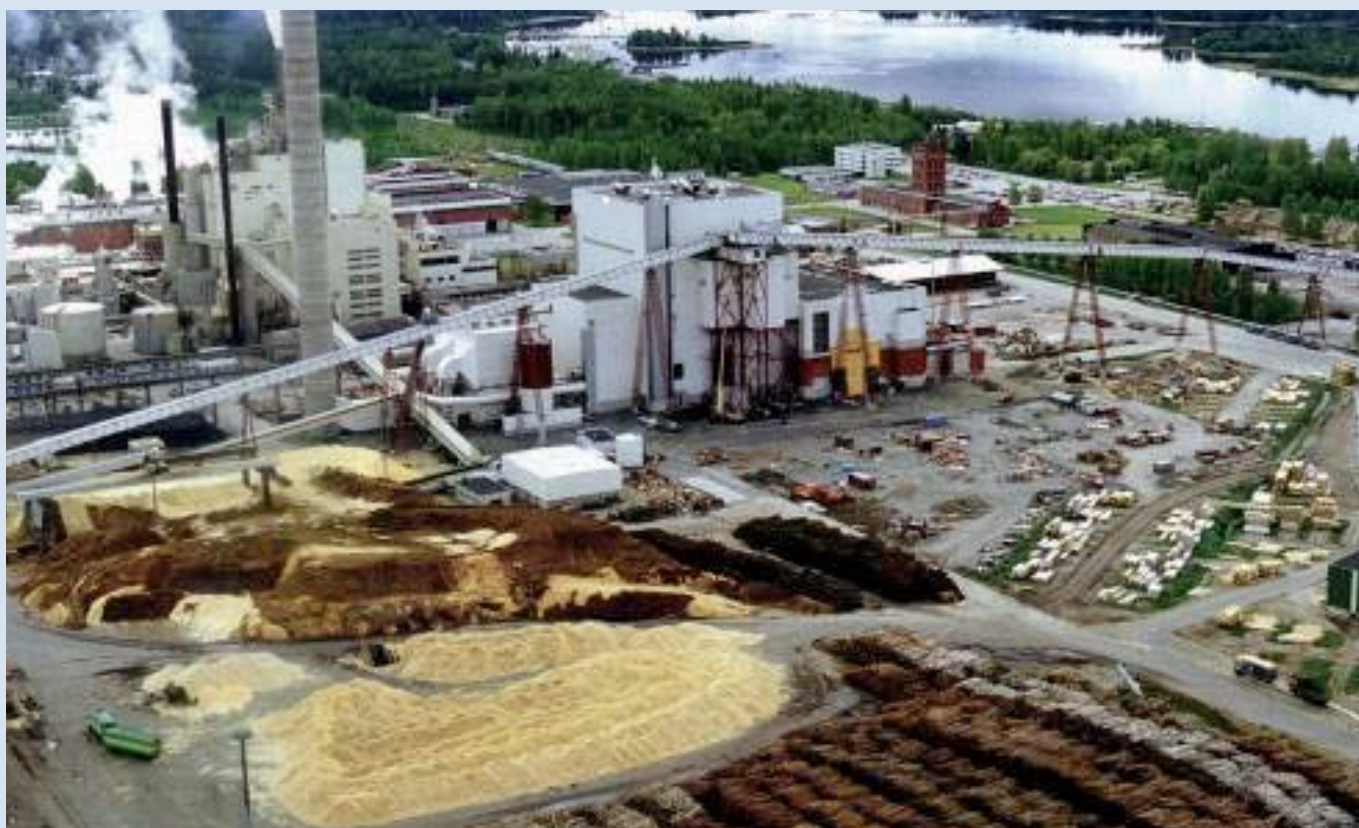
Figure 3.3: Alholmens Kraft Power Plant
