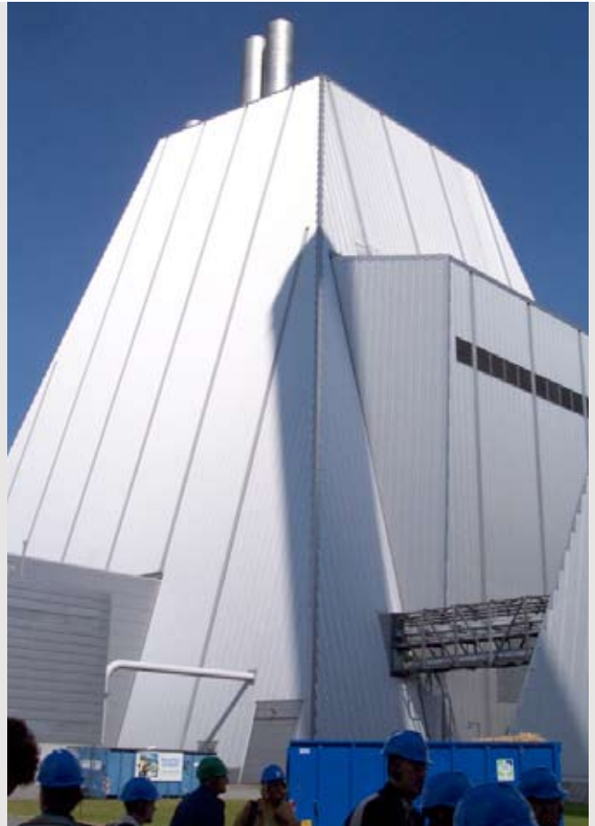
Figure 5.8: Avedore 2 Cogeneration Power Plant
