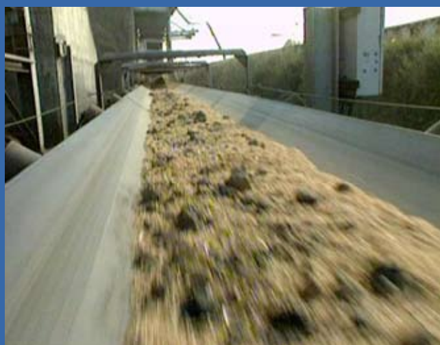
Figure 5.7: Wood Waste on Coal Conveyor Belt at Wallerawang Power Station
