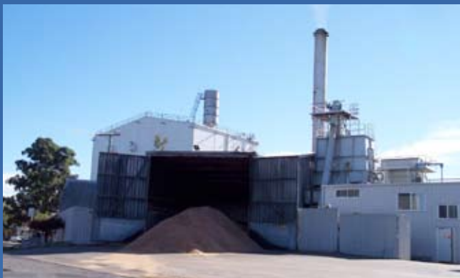
Figure 2.8: Bega Cheese Boiler House and Fuel Storage
