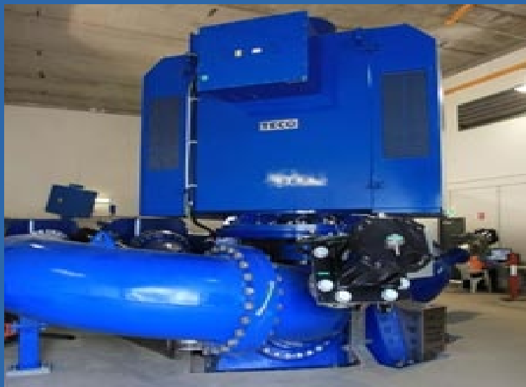
Figure 8: Sugarloaf mini hydro (Melbourne Water, 2010)
