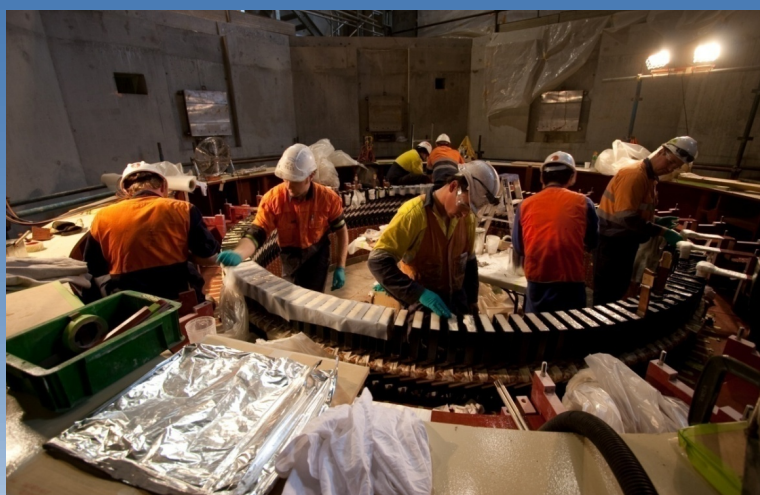
Figure 9: Bogong Power station construction - turbine inspection
