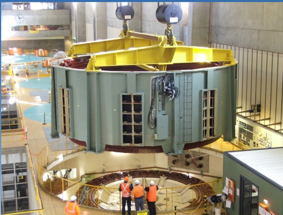
Figure 5 Stator lift (249 tonne) at Tumut 3
