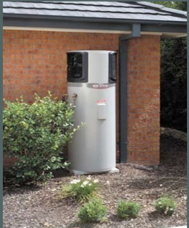
Figure 3b: Heat Pump installation
