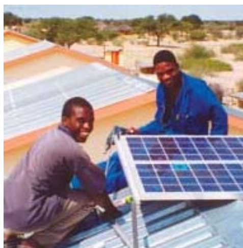
Installation of Solar Array
