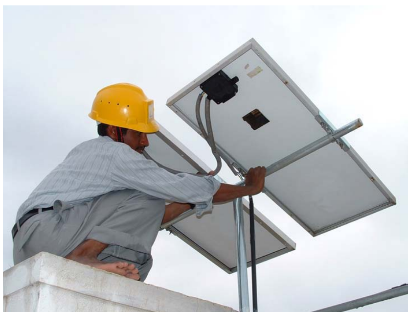
Panel Installation SELCO
