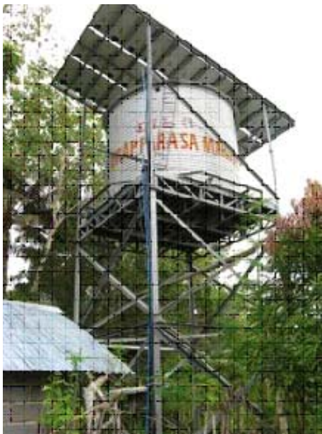
The dysfunctional 2.7kW solar water pumping system in Matarinao
