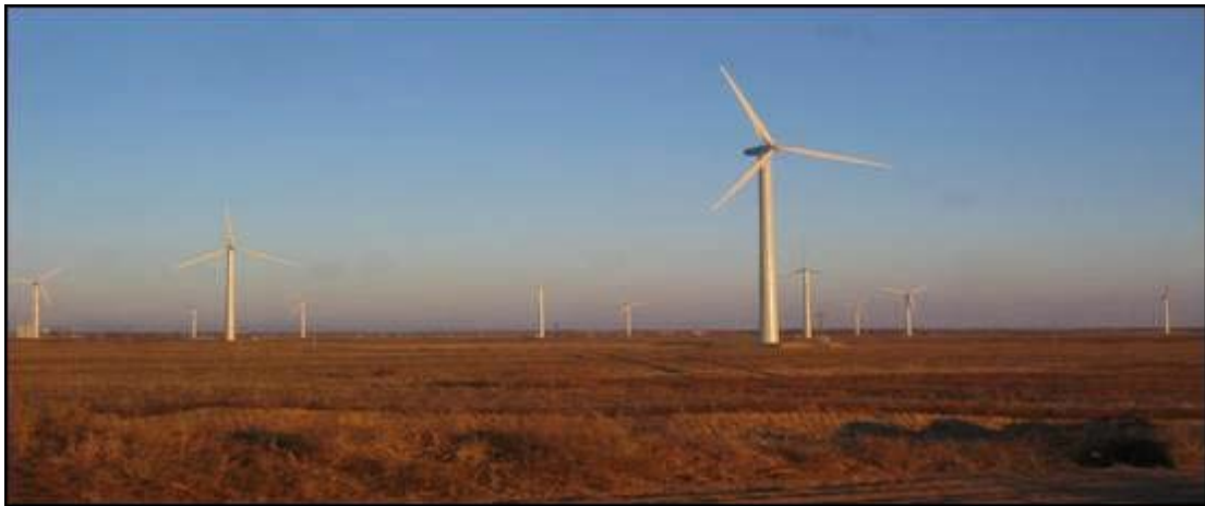
Figure 3: Shuangliao Wind Farm
